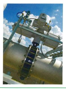
benefits of Rotork IQ intelligent electric actuation technologies, facilitating remote supervision with a high level of asset management encompassing accurate control, monitoring and alarm signalling, operational data logging and diagnostics. The ESD function can be configured to operate on loss of mains power or control signal, with additional options including a second, independent ESD circuit and an ESD manual reset also available.
